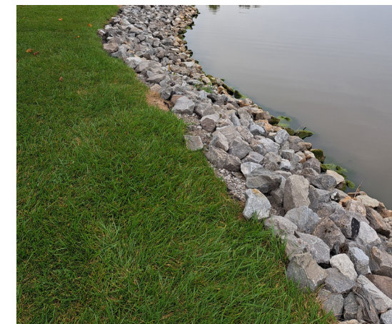
(Photos of shoreline with "riprap" installed)
